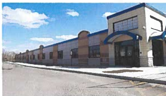
JOHN F. KENNEDY ELEMENTARY SCHOOL
