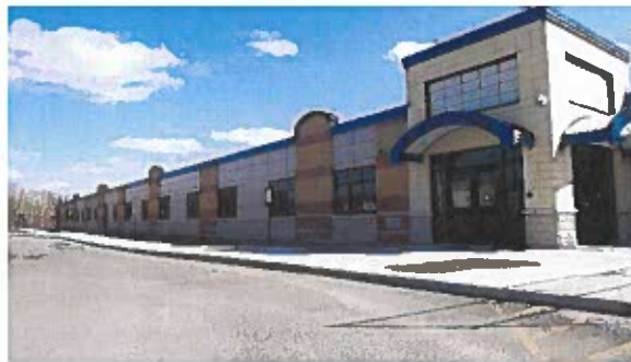
JOHN F. KENNEDY ELEMENTARY SCHOOL
