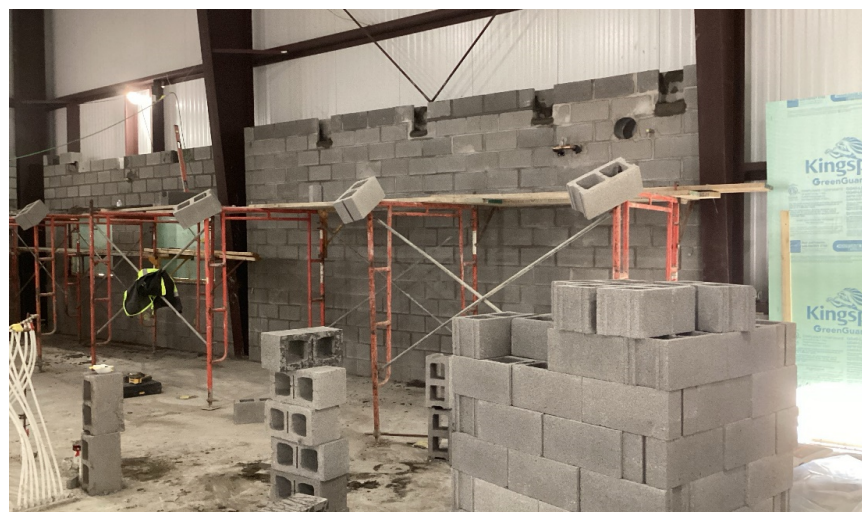
Interior Wall Construction at New Transportation Facility
