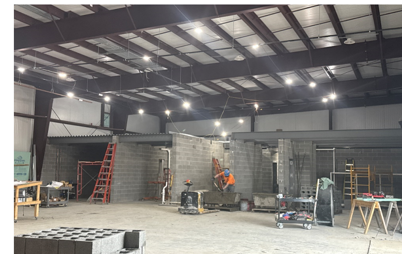
Construction of Office Space at Transportation Facility
