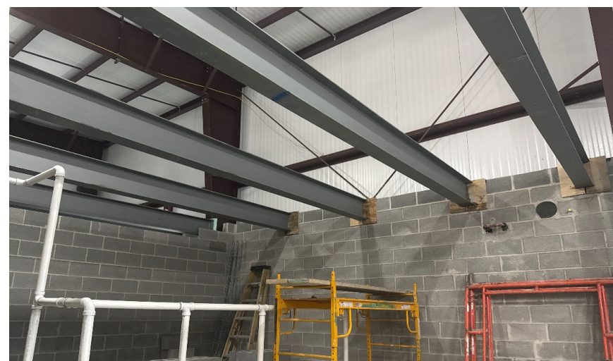
Second Floor Deck Framing at Transportation Facility
