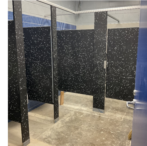
Dome Hockey Locker Room Toilet Room
