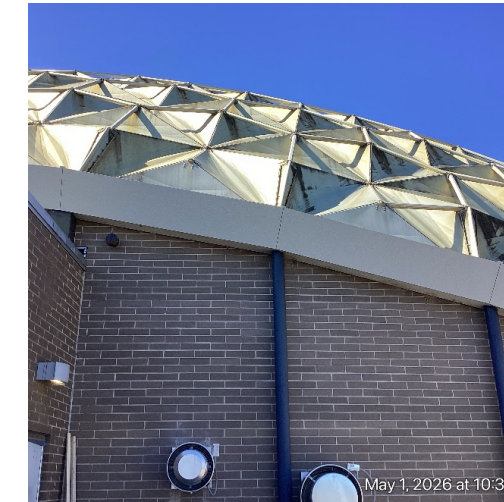
Gutter Fascia at the Dome
