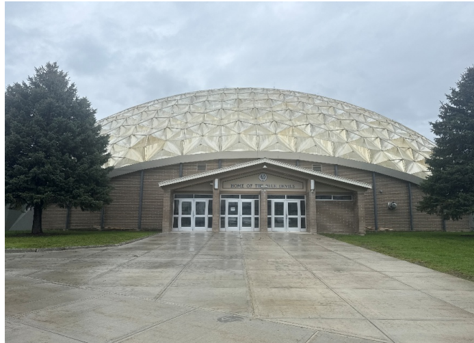
Gutter Fascia at the Dome
