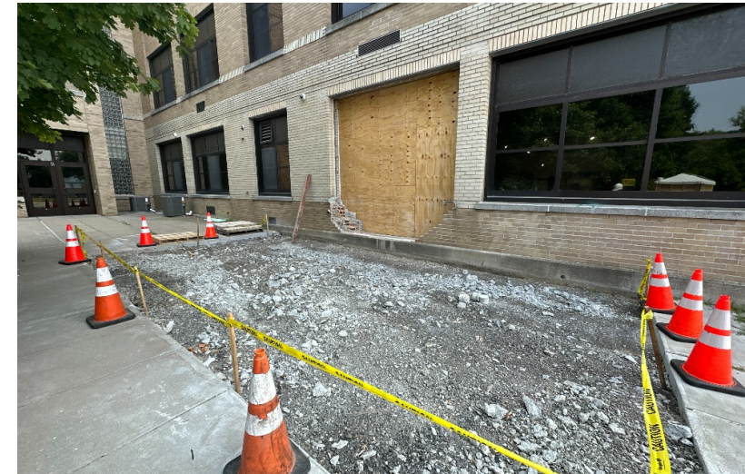
Opening for New Overhead Door at Create Room
