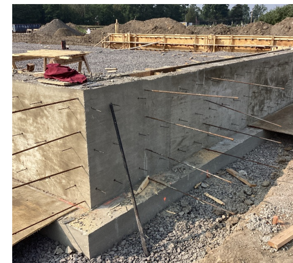
New Transportation Facility Foundations
