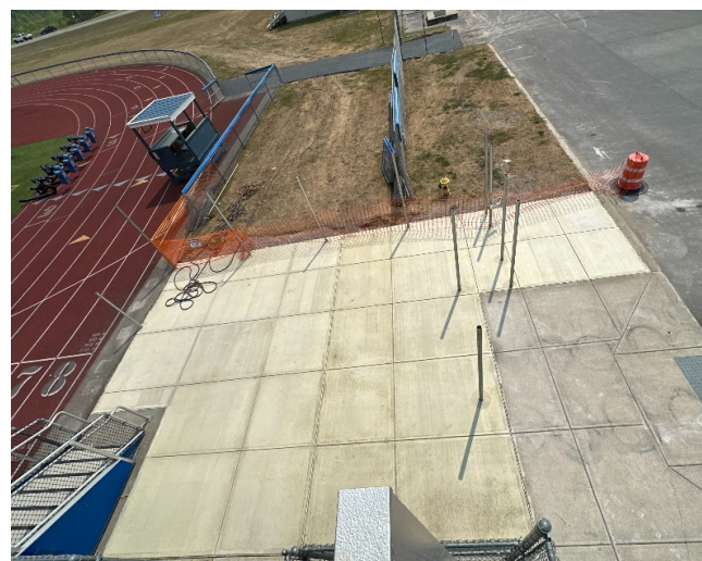
Concrete Pad and Fence Posts for New Grandstand Ramp
