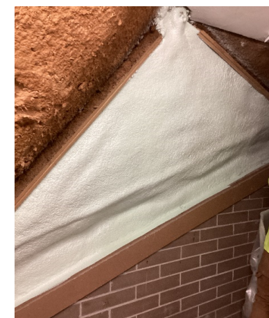
Sprayfoam Insulation Test Patch for Golden Dome Roof
